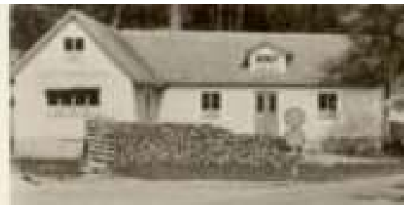
CLEO RAKKLINGA house, Ballingslöv
